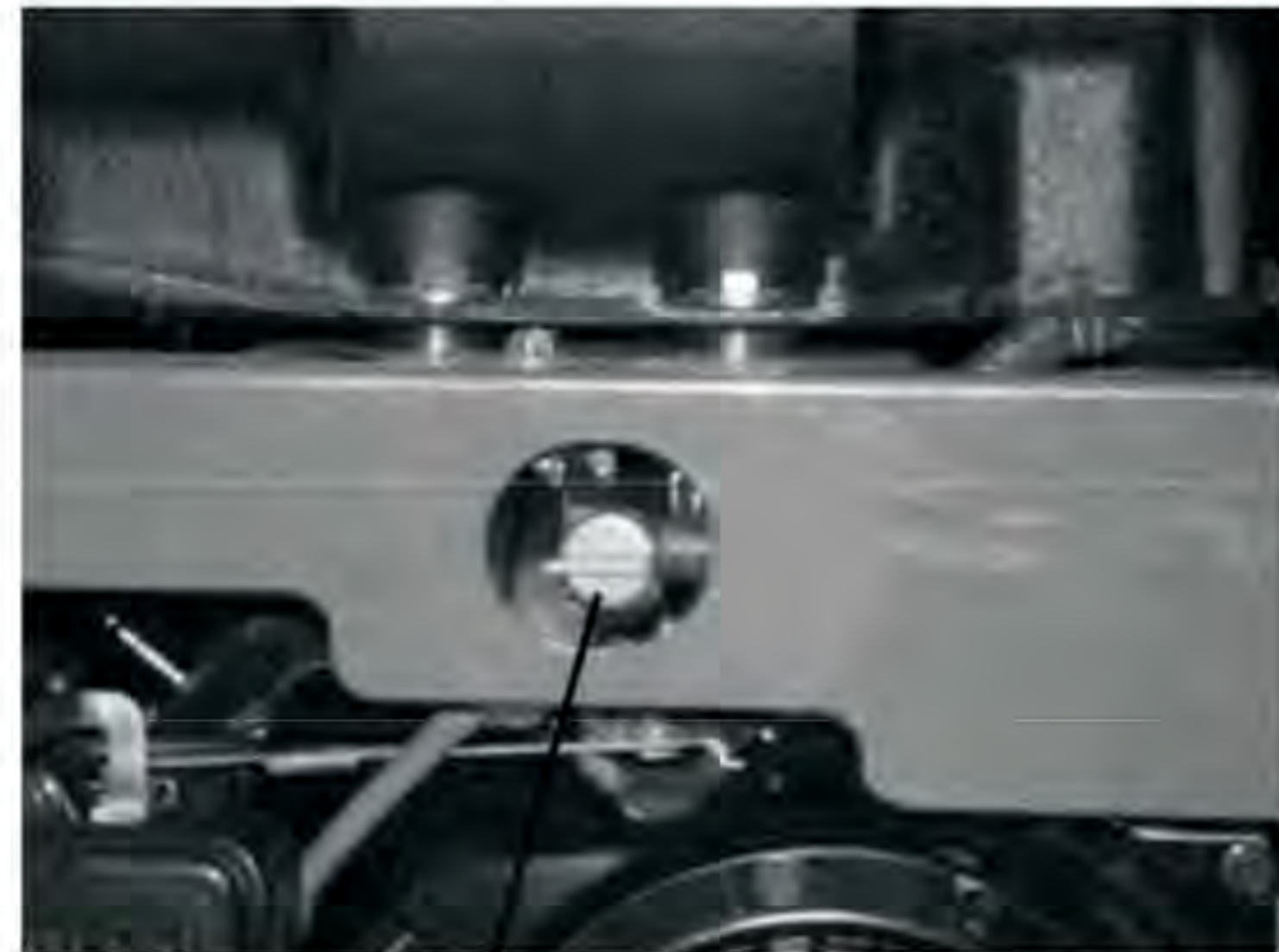
Fuel valve (OFF)
